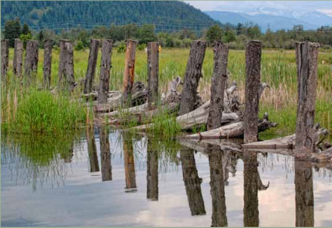
Above: As part of the Pack River Delta Restoration Project, root wad roughness structures (such as the one shown here) were constructed to slow annual flood waters from the Pack River and to trap the sediments the flood waters carry before they can be carried into Lake Pend Oreille. Pilings were driven into the delta bed. Large logs with their root wad facing into the projected current were securely fastened to the pilings. Photo by Nancy Miller
