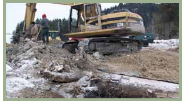
(Above) Heavy equipment at work during the construction of the islands in the Pack River Delta Restoration Project. Eight islands were constructed adding about 24 acres to the wetlands found in the delta.
