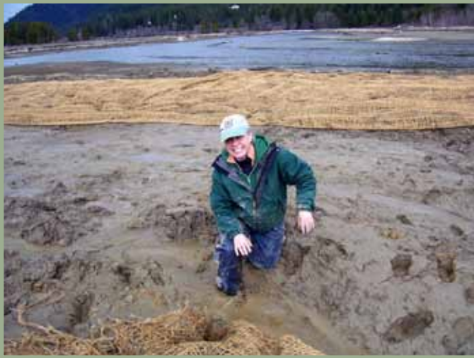
(Above) Kathy Cousins (IDFG) securing matting to protect the newly constructed islands from erosion during the Pack River Delta Restoration Project. Kathy will talk about this project and its application to restoration projects within the Clark Fork River delta during the annual meeting.
